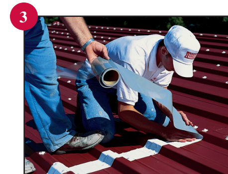
Treating the horizontal seams with Butyl tape
