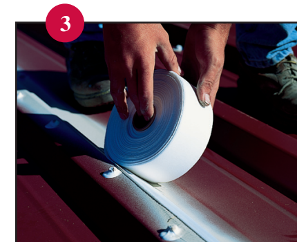
Treating the vertical seams with Spunflex fabric
